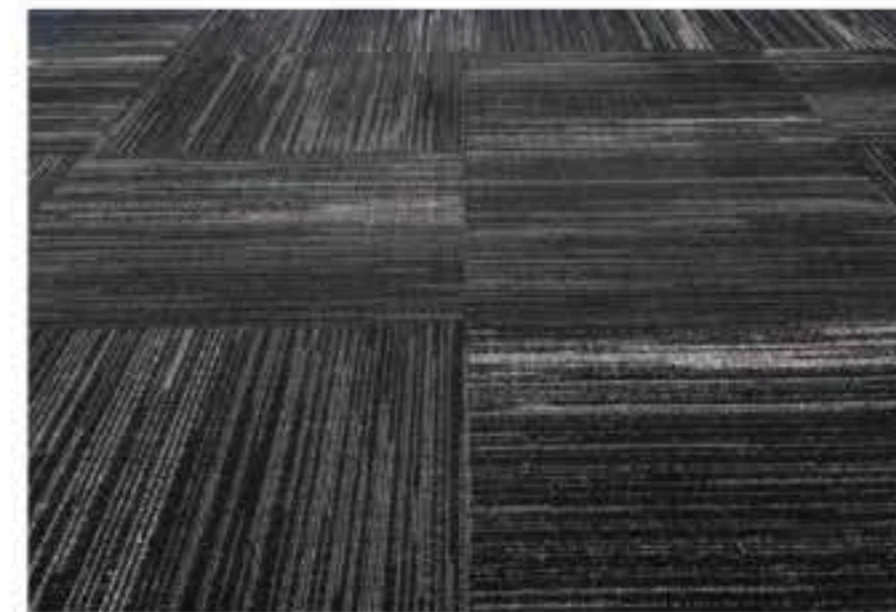
These 610 x 610-mm (24 x 24-in.) carpet tiles employ the 'random' installation method.
